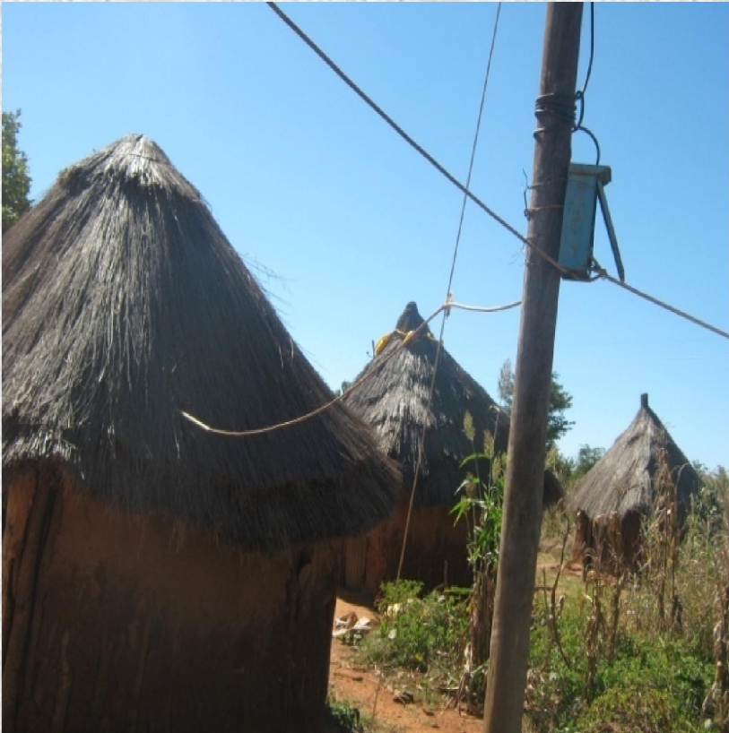
Pictures showing dangerous connections at farms
