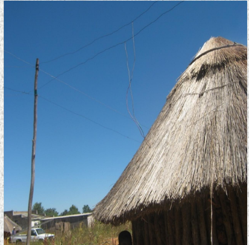
Pictures showing dangerous connections at farms
