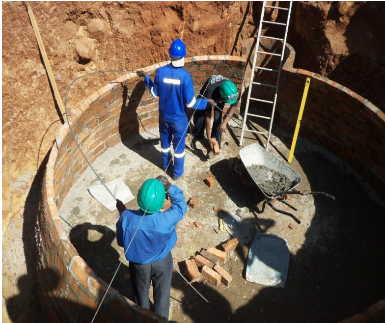
20m 3 Biogas Digester construction at Chibhero
