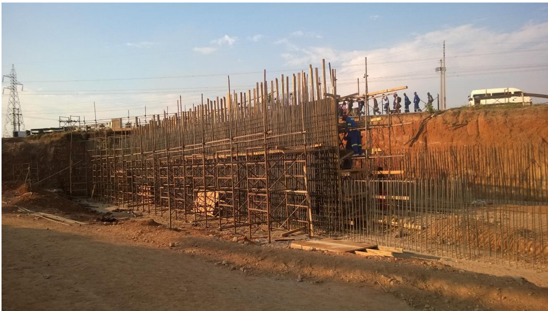
Mabvuku road over rail bridge
