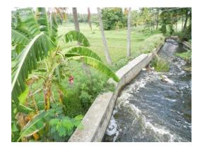
The SHEFROL plant was set up to remedy this civic problem. Every day, grey water (house-hold sewage) from 38 houses is fed into the plant that has a capacity of 10,000 litres. Costing only around ₹ 15,000, the plant consists of a sedimentation tank and channels created by sand bags placed in pits. This is covered by a non-permeable sheet that ensures wastewater does not seep into the ground as aquatic plants grow on top of it.
