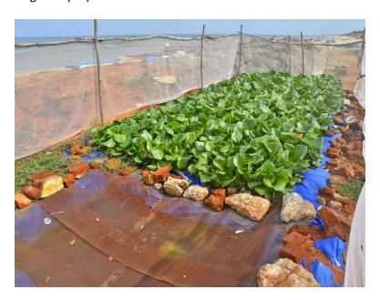
In 2005, Prof. Abbasi was working to develop an eco-friendly, inexpensive, and simple technology for waste water treatment when he came up with the idea of SHEFROL (which stands for sheet flow root level). With the help of university colleagues, S Gajalakshmi and Tasneem Abbasi, he carried out several experiments to fine tune the technology before setting up a pilot plant on the university campus.
