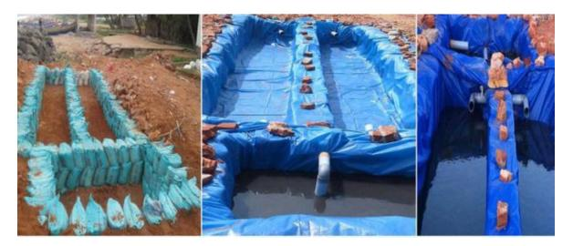
What also makes it a great option for villages, colonies or even large suburbs is the fact that it makes use of gravity and the topography, thus doing away with the requirement of pumping water. A small difference in fluid head between the inlet and outlet guarantees the constant flow of water in and out of the system.
