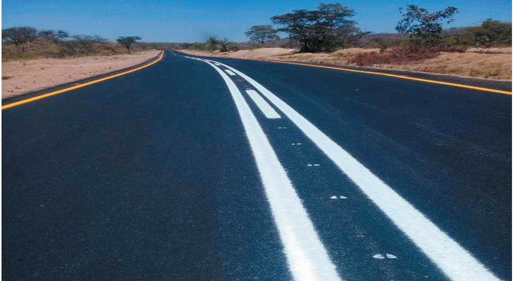
Completed section of the Bindura-Matepatepa Road
