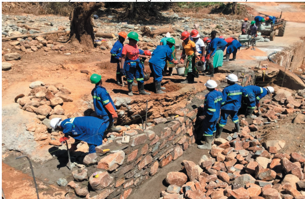
Mhakwe Causeway reconstruction in progress (Chimanimani District)
