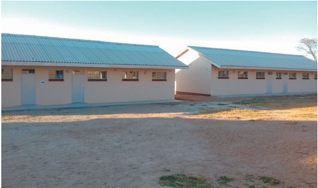
Tavoy Secondary School in Hurungwe – Mashonaland West
