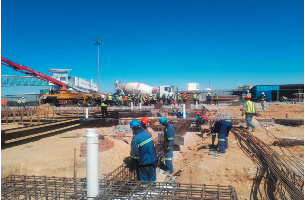
Work on foundations for terminal building extension
