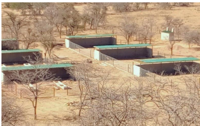
The Goat Holding Centre at Matopos Research Station is nearing completion. This formal goat aggregation facility will ensure that off-takers are able to access large volumes of goats at competitive prices.
