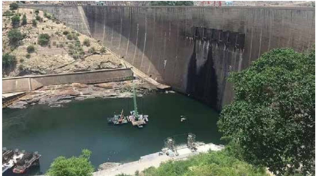
Caption: Kariba Dam wall renovations to the pool below, January 2020. @ JonGT/CC4.0
