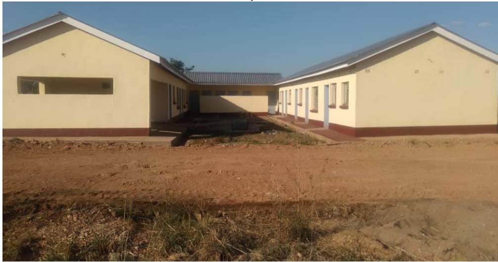
Ward 16 clinic almost comple and now fenced
