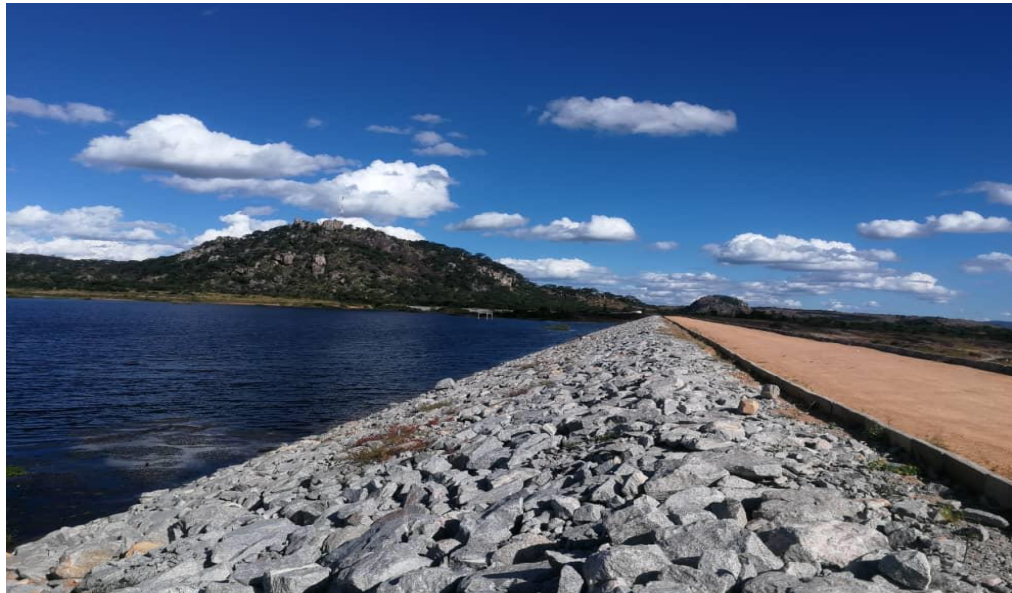
Newly Commissioned Muchekeranwa Dam
