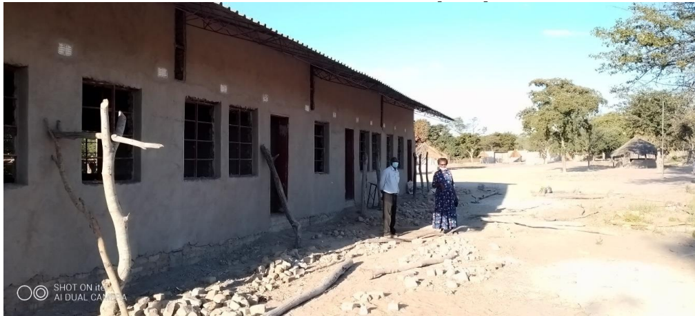
Classroom block under construction in Nyaminyami
