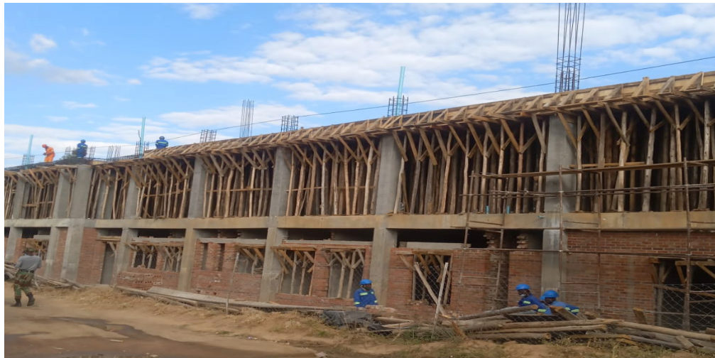
Ongoing works at Manyame VVIP hospital
