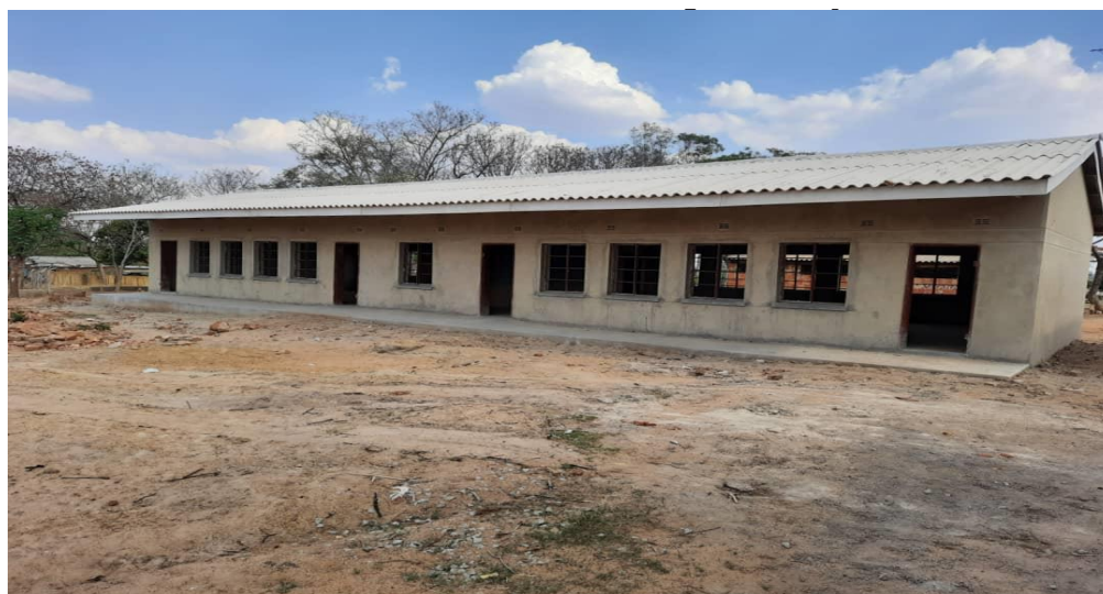
Construction of 1X2 Classroom Block at Raffingora Primary School
