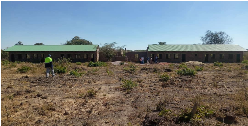
Two classroom blocks for Chidobera Primary School
