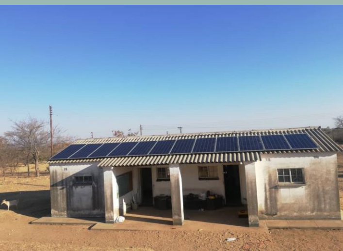
Rehabilitation of AHMCs in progress
